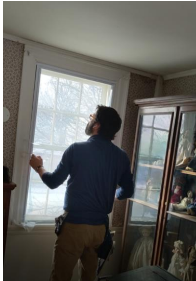
UV-blocking Film Installed on Windows.
